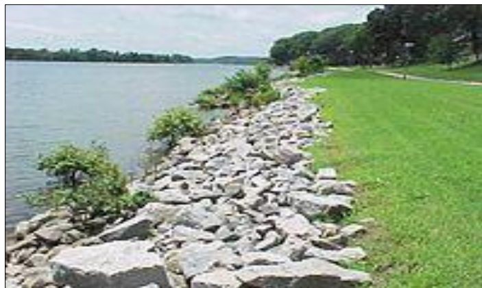
Figure 5 Riprap along Atlas Cove, Lagos, source field work 2012
